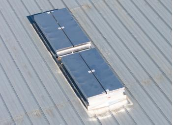
plans for NoDa Brewing included sprinkler activation, but fire protection officials mandated the design include the smoke vents.
